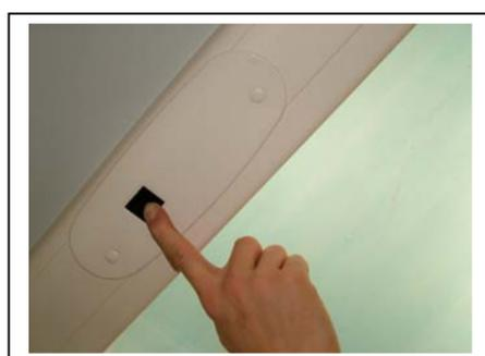
Push the button so long that the desired position is reached or the electrical motor switches off.
